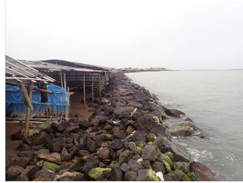
Protection Measure (Rock Fill)
