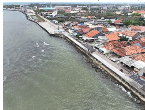
Coastal Protection at Urban Area (Line Protection)
