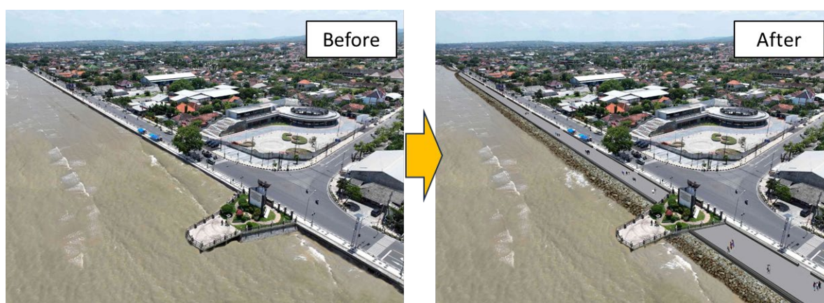
Figure 4.4 Image of Before- and After-Implementation of Revetment Type-1 (T-b)
