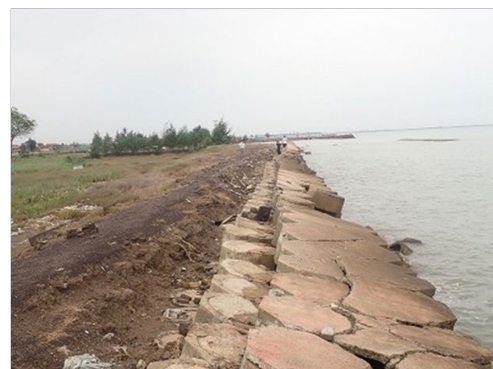
Collapse of Seawall due to further erosion
