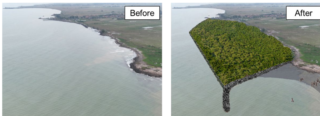
Figure 13.3.10 Implementation Image of Mangrove Plantation and Breakwater for Mangrove Protection (Area-II, S-4a)
