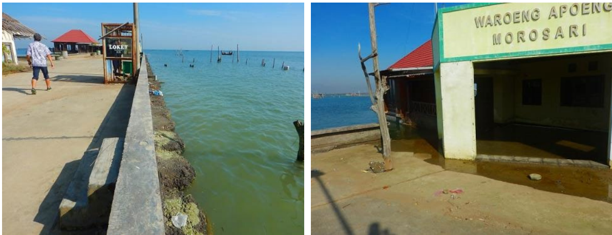
Photo 2 Restaurant and Surrounding Seawalls at the Survey Site
