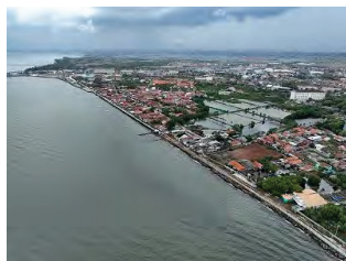
Coastal Protection at Urban Area (Line Protection)
