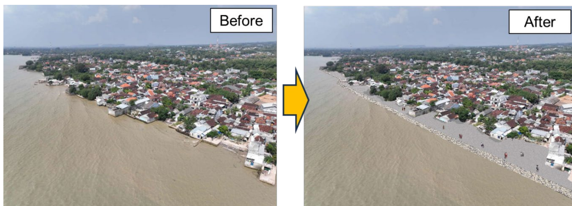
Figure 13.3.15 Image of Before-and After-Implementation of Type-2 Revetment in Tuban (T-c)
