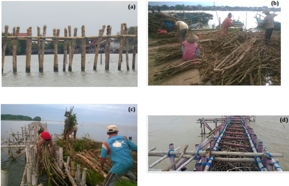
Figure 2.7.7 Case-1: Permeable Dams Installed as Hybrid Engineering (HE)
