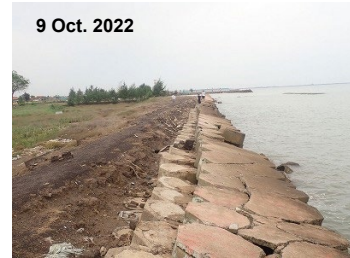
Collapse of Seawall due to further erosion (P1)
