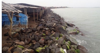
Protection Measure using Rock Fill (P1)
