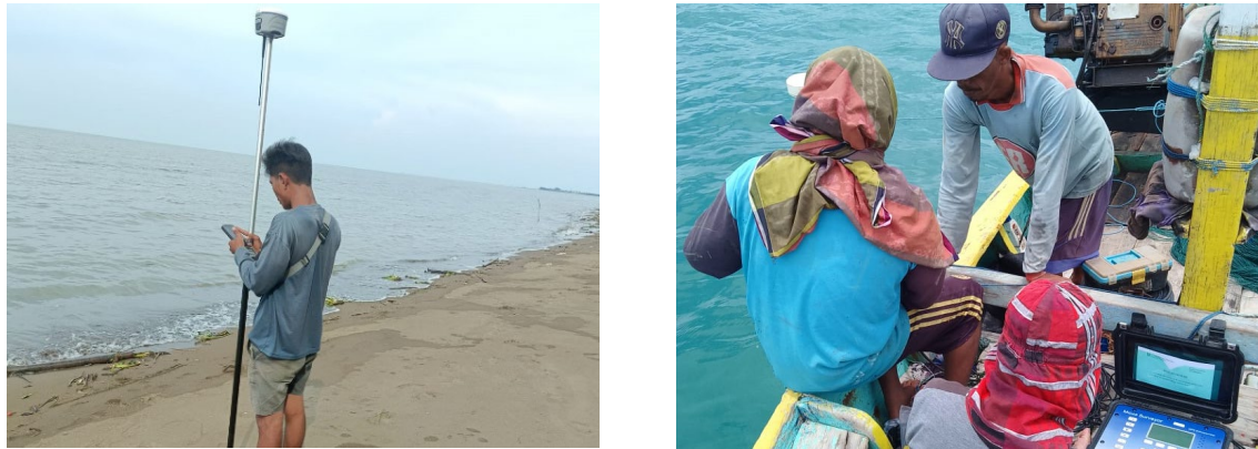
Figure 3.1.3 Survey Work (Left: Topographic Survey, Right: Bathymetric Survey)
