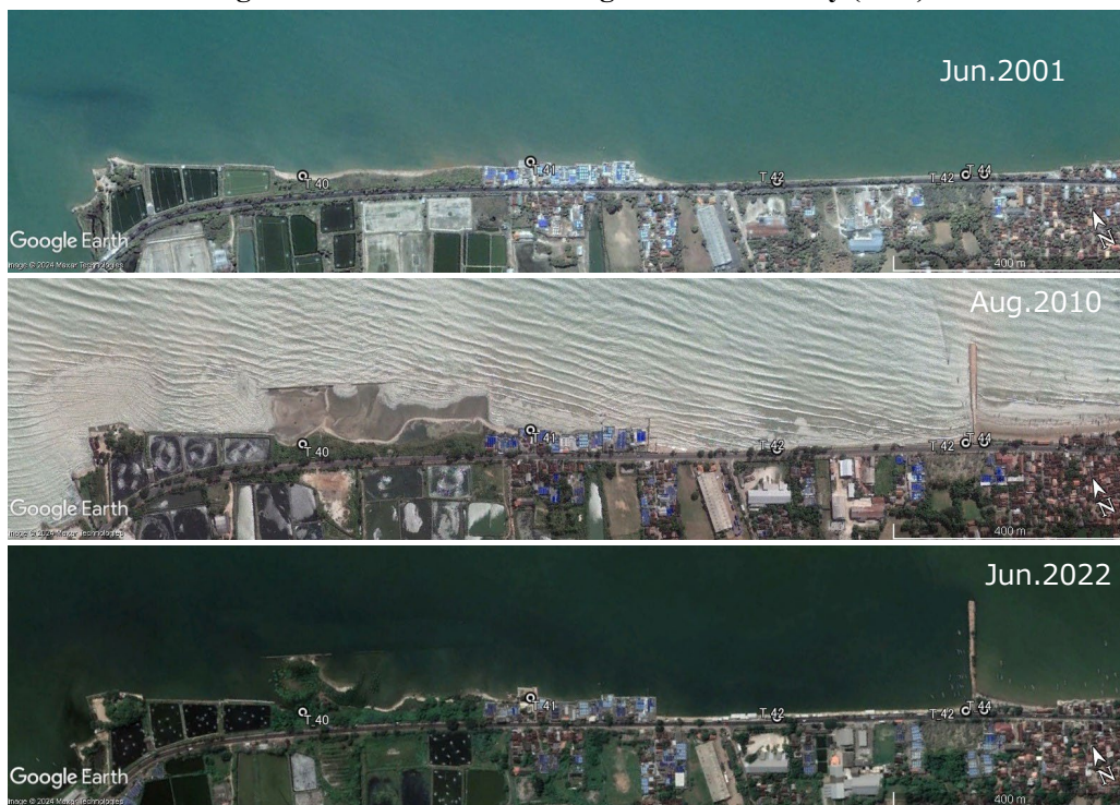
Figure 12.2.14 Shoreline Change Around the Offshore Breakwater and Jetty (No.6)
