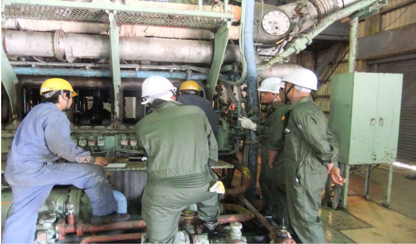
Crankshaft Deflection measurement before disassembly
