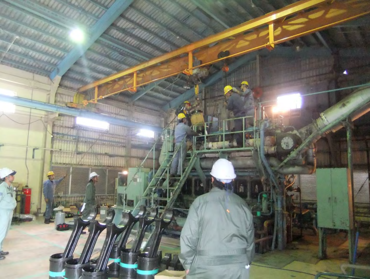
Cylinder Liner extraction
