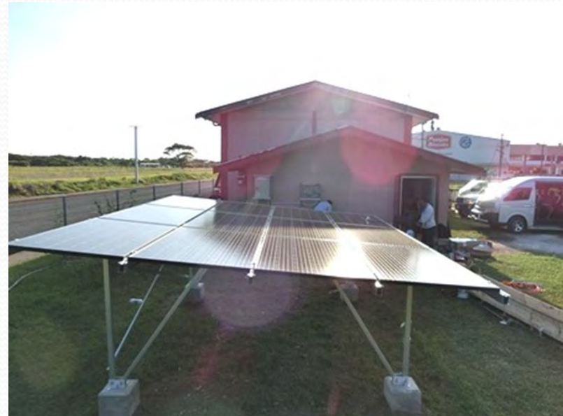
RE Training (construction of 3.5 kW solar power facility)
