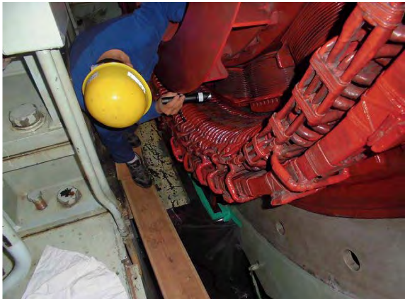
• Generator Checking inside 2
