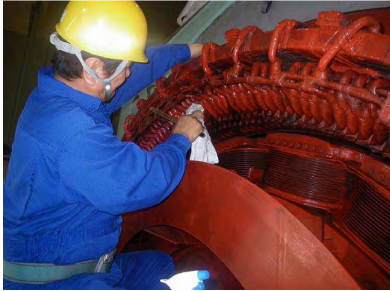
13. Generator Cleaning picture • Cleaning inside 1
