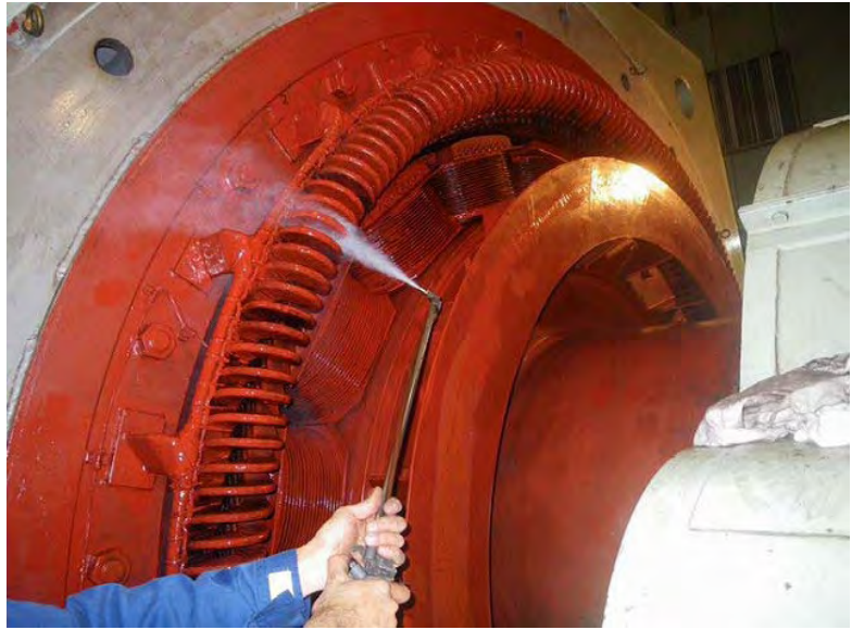
12. Generator Washing photo ▪ Washing with an electrical cleaning agent
