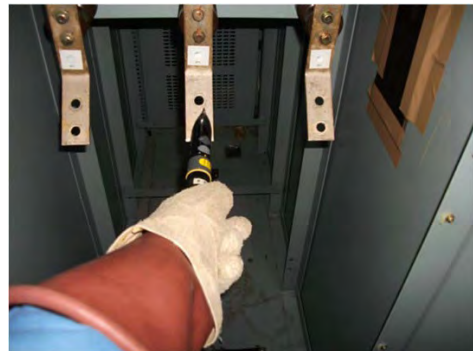
Electroscope work
