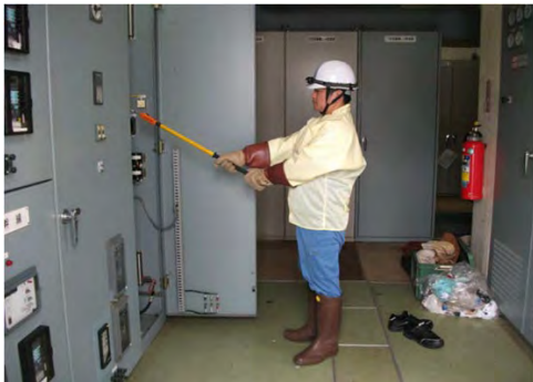
Electroscope work
