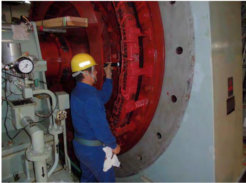
11. Internal inspection Air blow picture • Generator Checking inside 1
