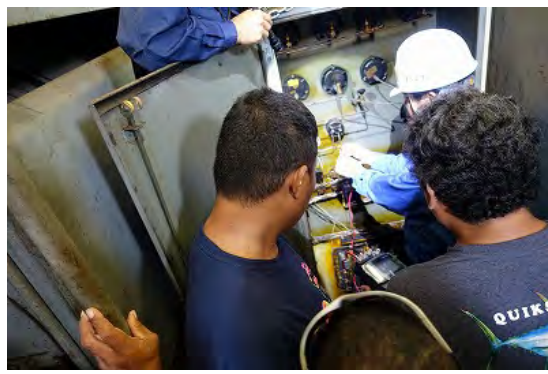
06-Inspection of analog meters, Loop test
