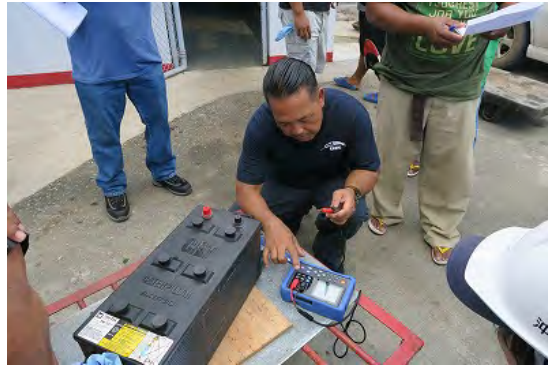
04-Inspection of batteries(internal resistance)
