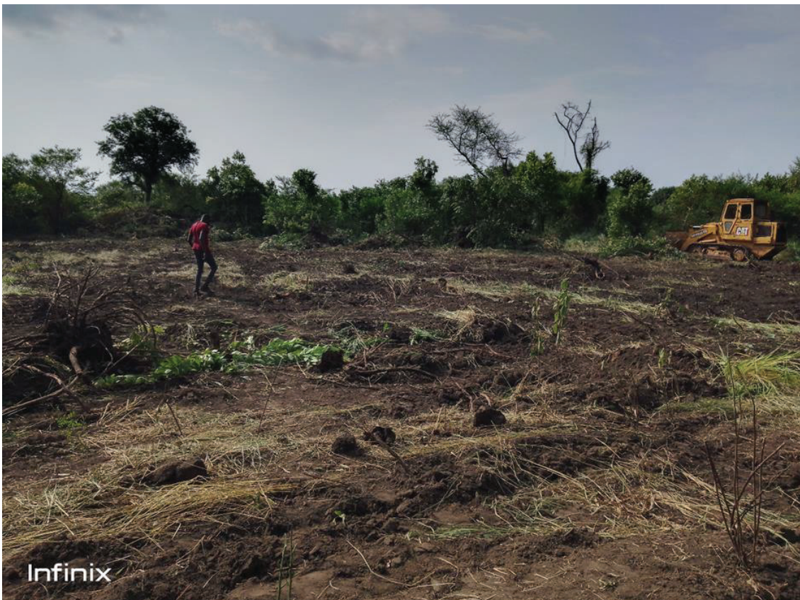
Above; Bush clearing using bulldozer.
