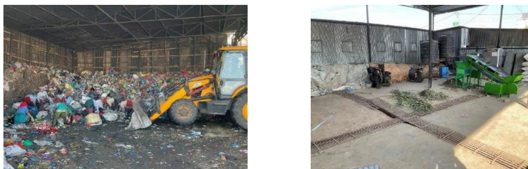
Figure 4-12 Recyclable Sorting and Composting Facility by Shirjanship Sewa Pvt. Ltd.
