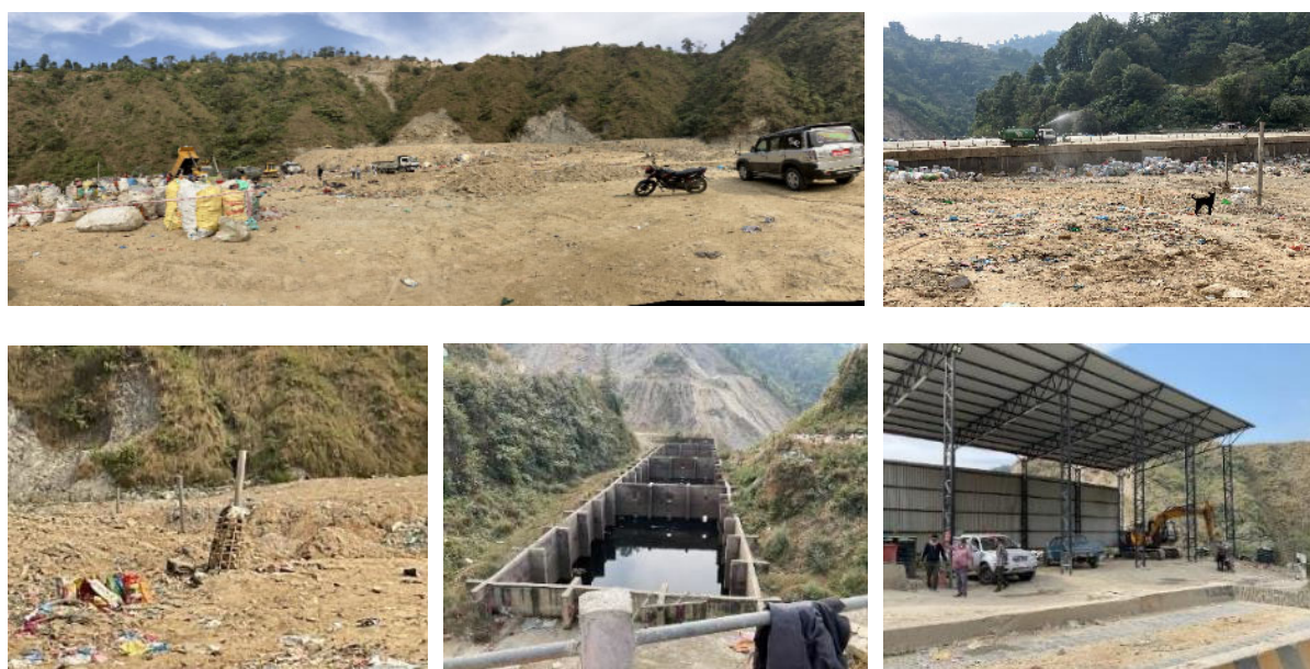
Figure 3-24 Summary of Facilities at the Banchare Danda Landfill Site
