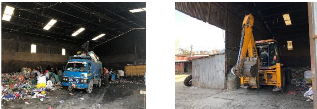
Figure 3-13 NEPCEMAC Pvt. Ltd.'s Transfer Station
