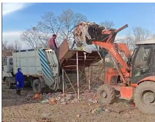
Loading waste on compactor
