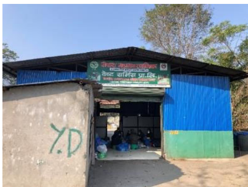
Front of treatment facility
