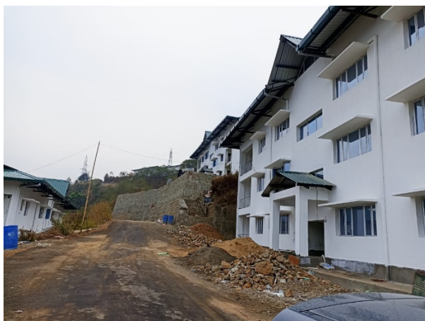
Exterior of 100-sqm Apartment
