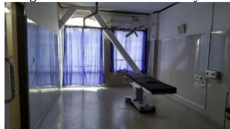
Operating Room under Construction
