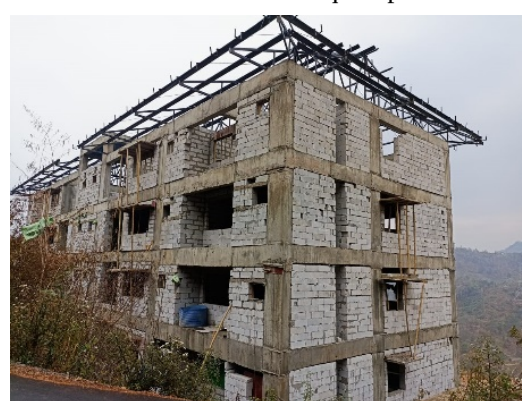
Exterior of 200-sqm Apartment
