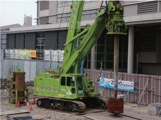
Earth drill machine image
