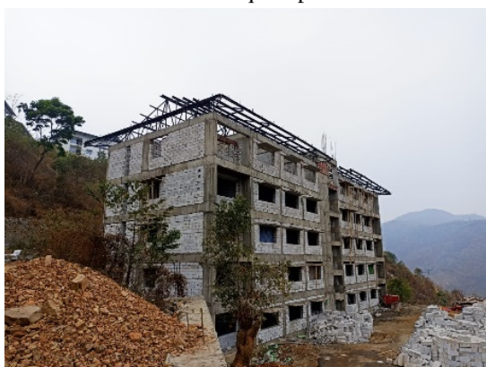
Exterior of 200-sqm Apartment
