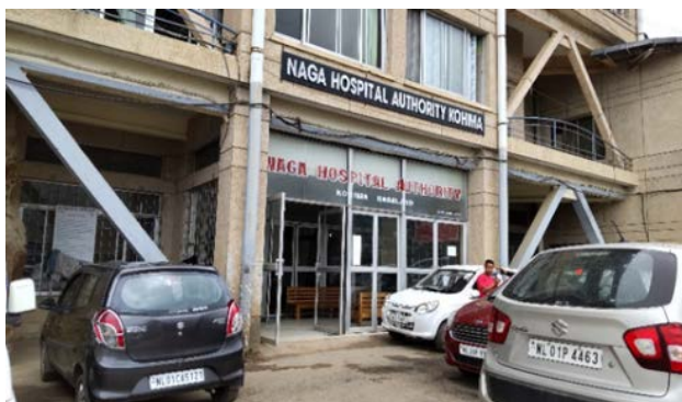
Entrance to the Central Treatment Building
