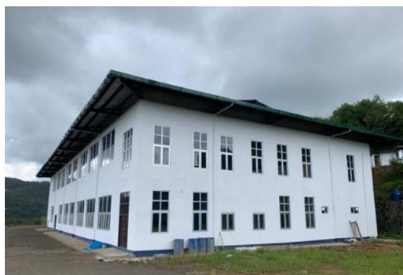
Exterior View from the North
