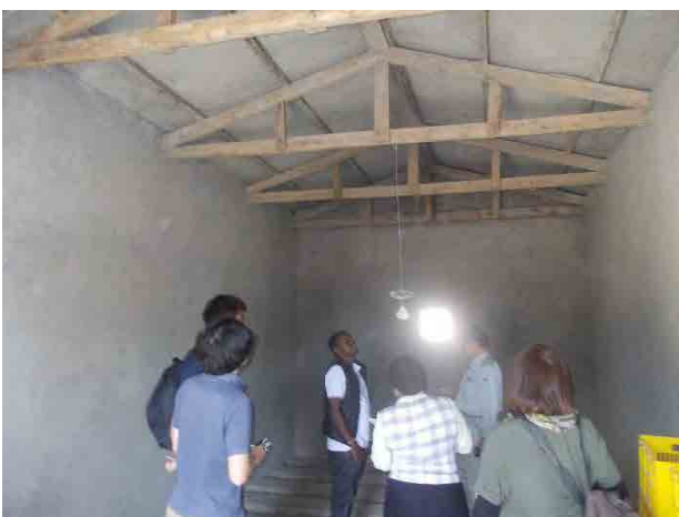
Potato-storage facility exterior (up) and interior (down).
