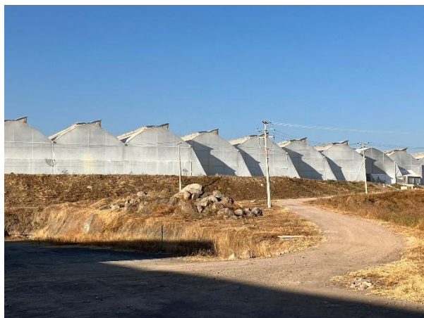
Vinyl greenhouses are deployed on a 30 ha site. The system is automatically controlled according to the indoor environment.
