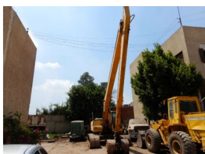
Long Arm Hydraulic Excavator (Active)
