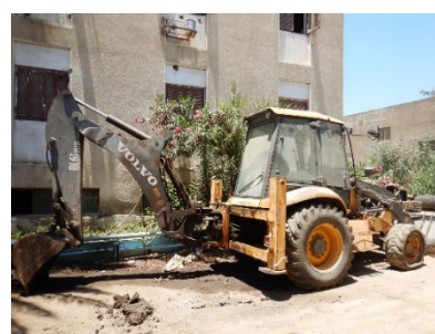
Backhoe Loader (Active)
