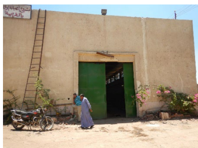
Outside View of Workshop
