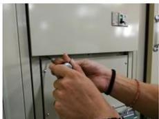
① Remove the 3 screws at the bottom of the Operation board
