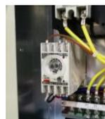
**Electric power controller** should be set at 100. You can increase/decrease the output of electric heater.
