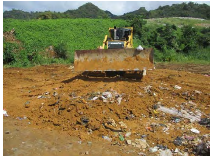
Soil cover with excavated soil on site
