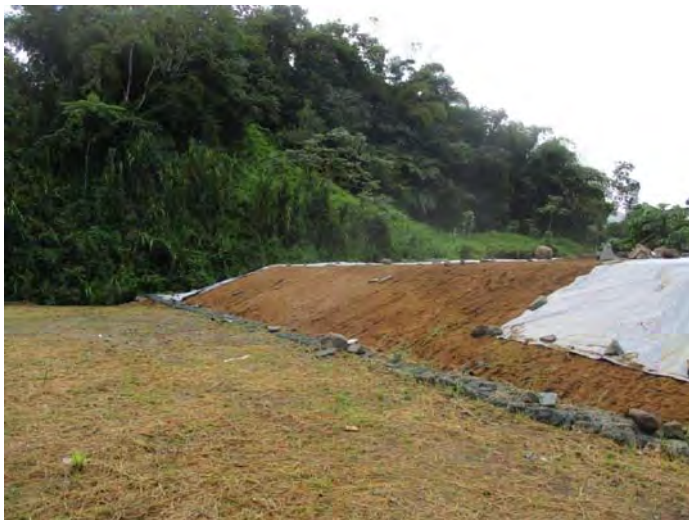
Embankment and adjacent ground
