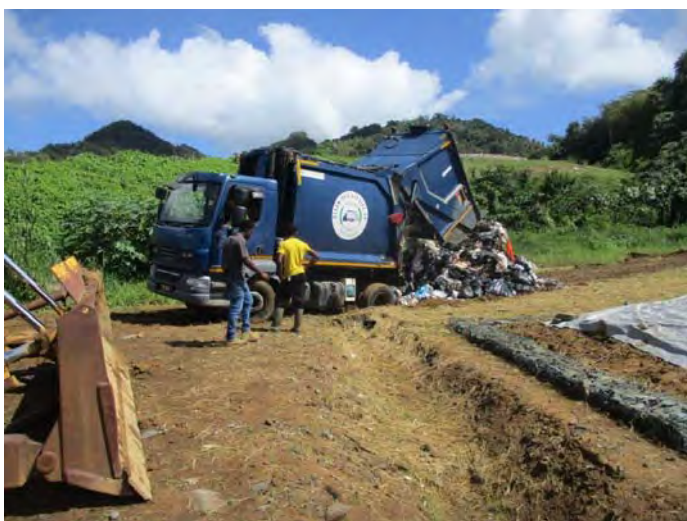
RCV tipping for the preparation of the first layer
