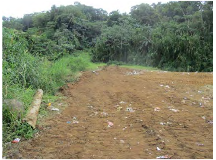
Access road was improved again
