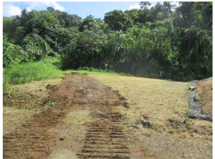
Access road and drainage
