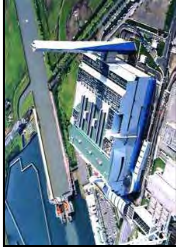
Shin-kouto incineration plant (capacity: 1,800t/d) (capacity of electricity generation: 50,000kW)
