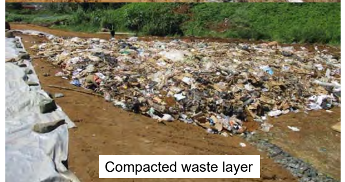
Compacted waste layer
