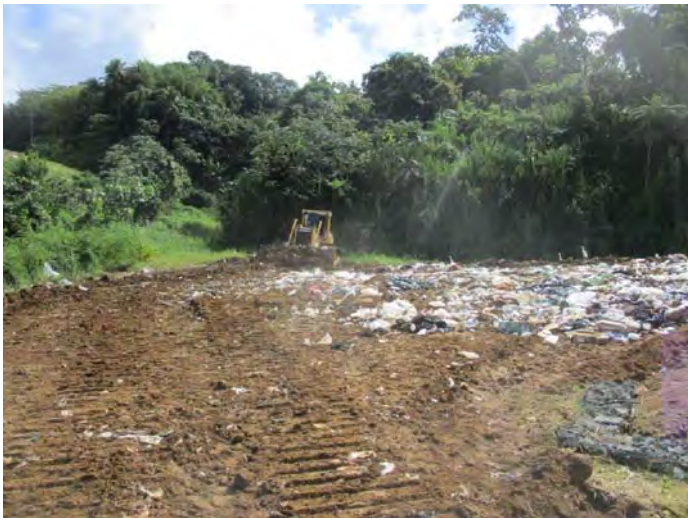
Soil cover with the existing ground soil
