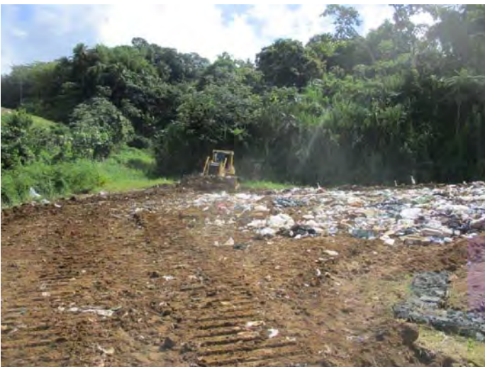
Soil cover with the existing ground soil
