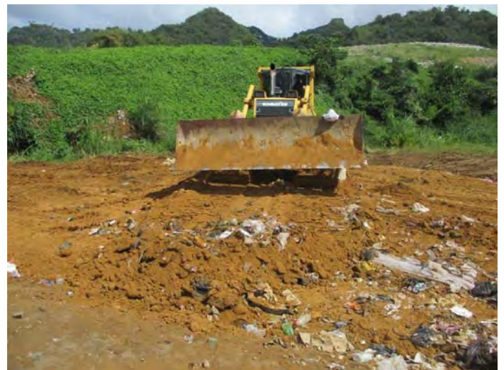
Soil cover with excavated soil on site
