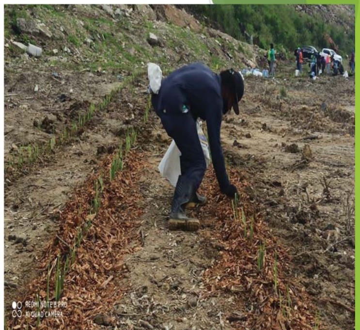
Planting of vetiver grass in the flashes west of the old landfill site
