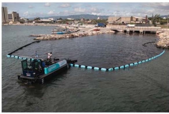
Debris is trapped by the Interceptor™ Barriers
