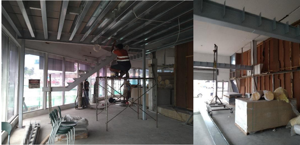
Figure3-2-15 : Example of using lightweight steel frames for partition walls and ceilings at a renovation site
