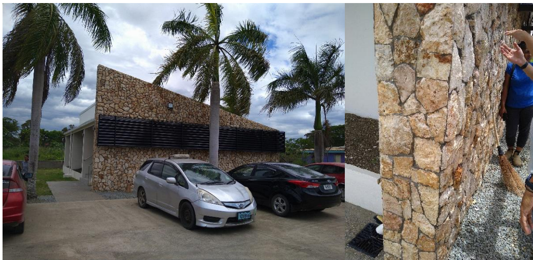
Figure3-2-14 : Example of construction using Fijian domestic stone and the Finish of its detail part.
