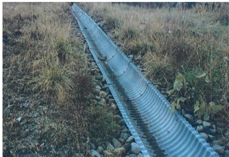
Corrugated pipe channel: Functions of the channel can be sustained even with ground deformation.
