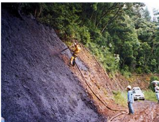
Photo 4. Spraying of soil
