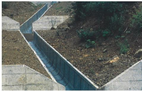
Corrugated flume pipe channel: For locations where flexibility in work needed such as landslide area, etc.
