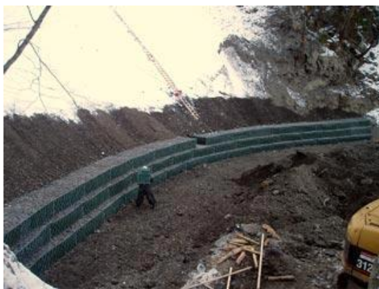
Figure 3-8 Material types of Retaining wall work: Gabion box retaining Work (left) and Log retaining work (right)
