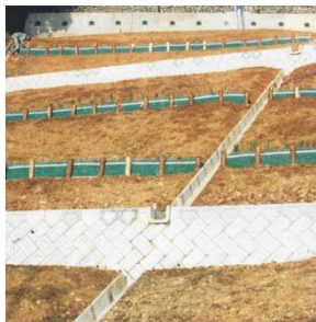
Precast concrete channel: Channel material is precast concrete and Easily procured.
