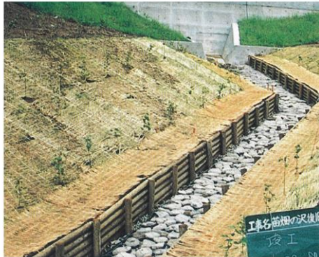
Wooden fence channel: It is compatible with vegetation work. Relatively low durable.
