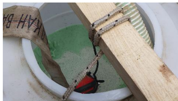
Photo 18. Installation of pumps in tanks
