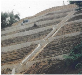
Wet masonry hillside channel: For locations with high volume constant water
