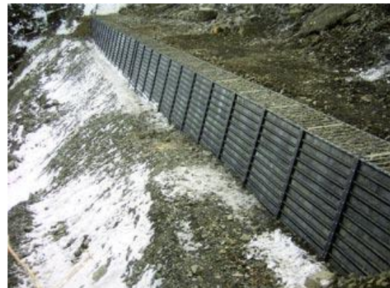
Figure 3-7 Material types of Retaining wall work: Wet masonry retaining work (left) and Steel frame retaining work
