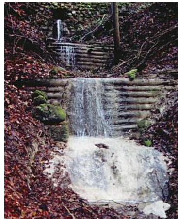
Figure 4-2 Small step check dams made of natural materials in North Macedonia
