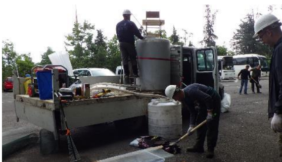
Photo 17. Equipment installation condition
