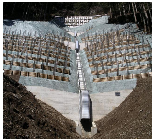
Figure 3-5 Retaining wall work combined with Fence work and Hillside channel work
