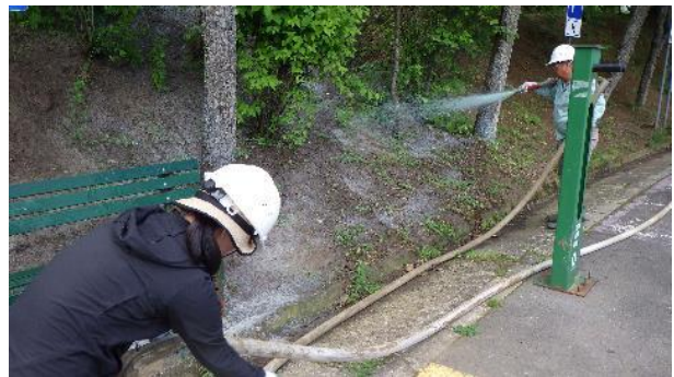
Photo 21. Nozzleman's assistant adjusting hose position
