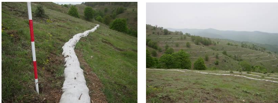
Photo 11: Robinia planting with terracing work in North Kodzalija
