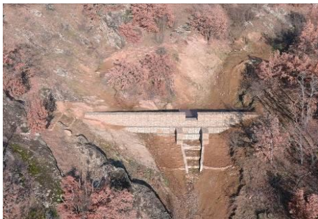
Photo 12: Gabion gully plug and terracing work in Lisiche site
