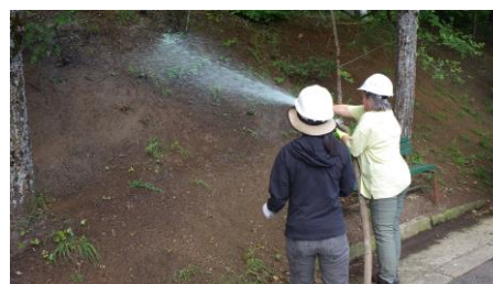
Photo 14: Demonstration of Hydro-seeding
