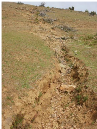
Photo 21: Place with advanced erosion, where installation of a gully plug is considered
