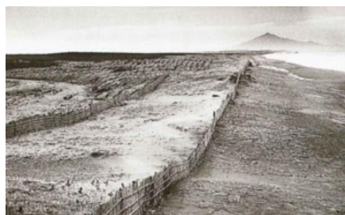
Fences to control and accumulate flying sand constructed in 1960
