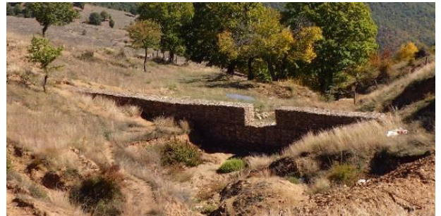
Figure 4-1 Gabion check dam in Lisiche and Radovish constructed and demonstrated in the Eco-DRR Project in North Macedonia
