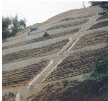
Wet masonry hillside channel: For locations with high volume constant water
