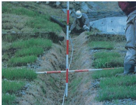
Sod covering channel: Suitable for gentle slopes with no constant water, low water discharge, no sediment movement and rich soil for sod to grow
