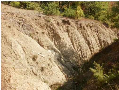
Photo 15: Place with advanced erosion, where installation of a gully plug is considered
