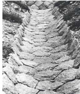
Wet masonry hillside channel: For locations with high volume constant water
