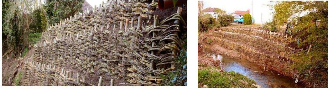
Figure 3-24 Fence works in North Macedonia, in Wicker woven fences
