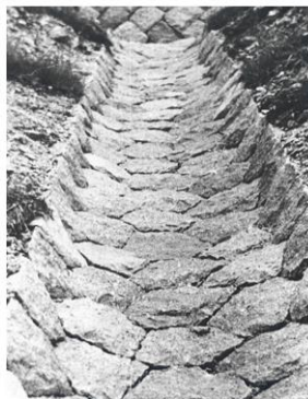
Dry masonry channel: For steep slopes without constant water
