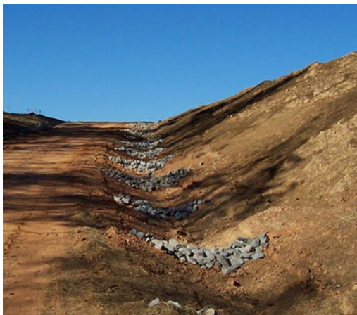
Figure 4-2 Small step check dams made of natural materials in North Macedonia
