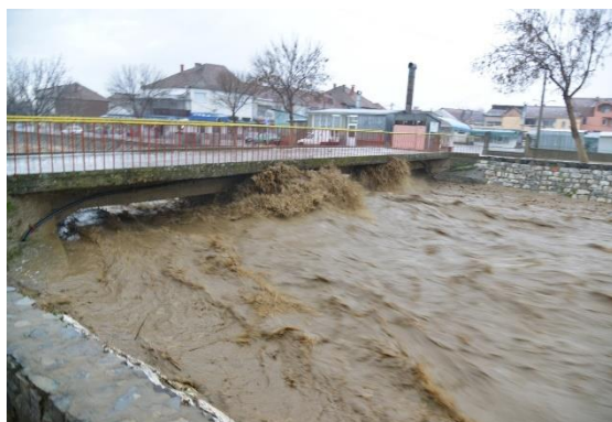
Photo 3: Radovishka River in flood in 2015
