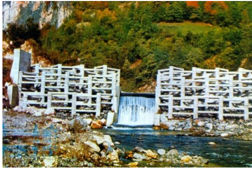
Figure 4-3 Classical Open type check dam in Tetovo (left) and Combination type check dam (right)
