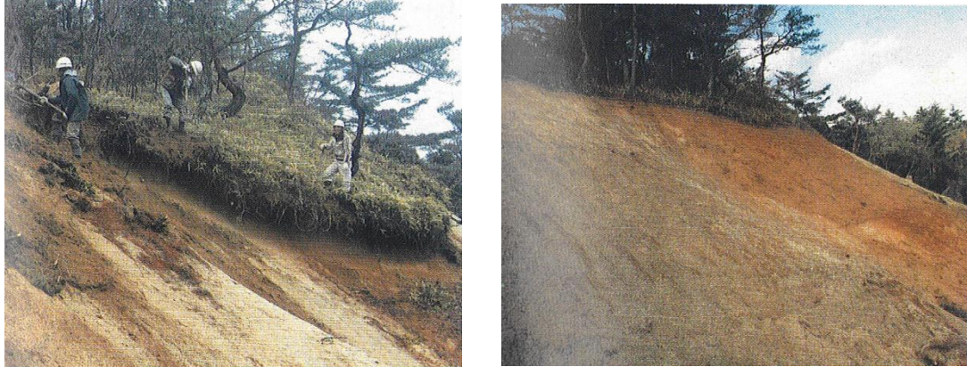
Figure 3-3 Grading work: work in progress (left) and after completion (right)
