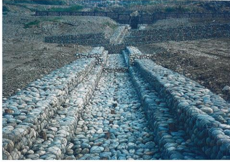
Gabion box channel: For locations with soft ground and little constant water
