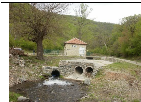
Photo 4: Ljubanci small hydropower facility (Forest compartment No 90)
