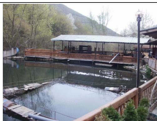
Photo 3: Ljubanci Village water abstraction facility (Forest compartment No 89)
