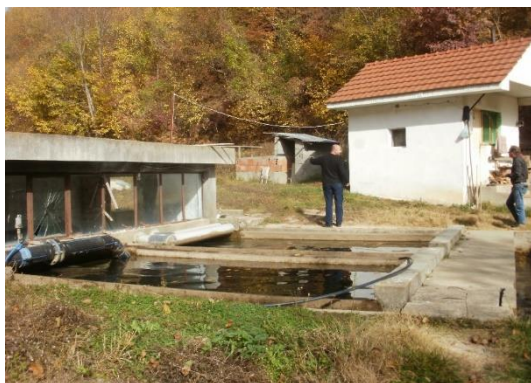
Photo 3: Water intake facility of Radovish Town
