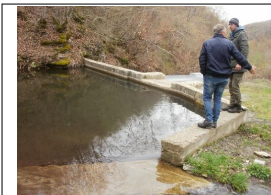
Photo 2: Kučevište village water abstraction facility (Forest compartment No 62)
