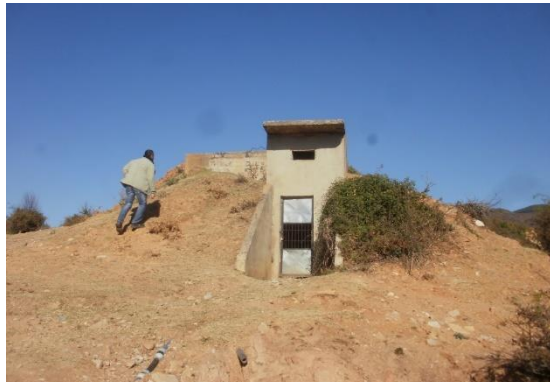
Photo 5: Water intake point of Kalauzlija and Shturovo Villages
