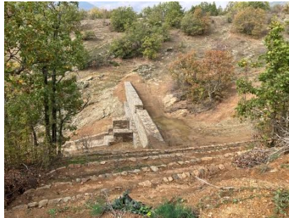
Photo 12: Gabion gully plug and terracing work in Lisiche site
