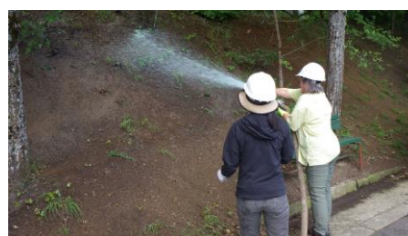
Photo 14: Demonstration of Hydro-seeding
