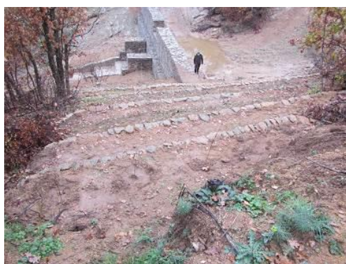
Photo 13: Tree planting with terracing work and micro water catchment work in Lisiche
