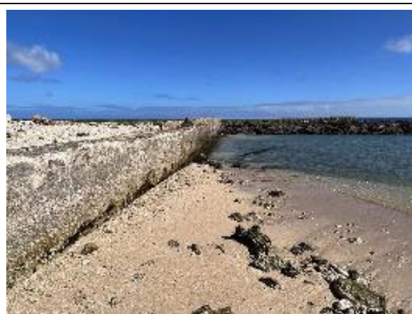
Photo 2.7.23 Concrete Block Quay of Old Port
