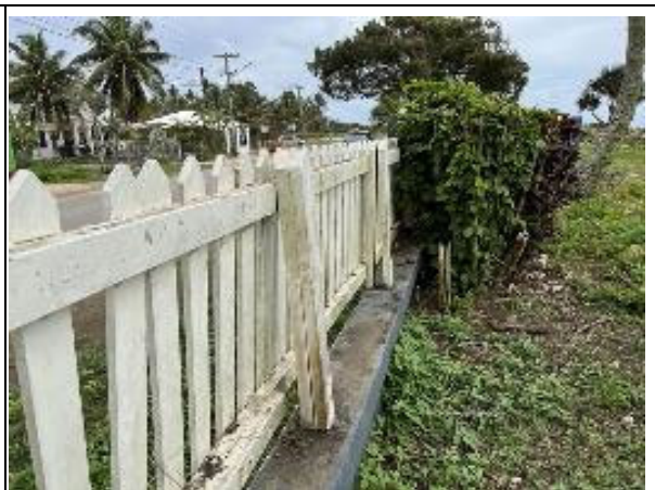
Photo 2.7.6 Fence Pushed back by Tsunami
