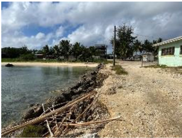
Photo 2.7.25 ①Masonry seawall of north wharf
