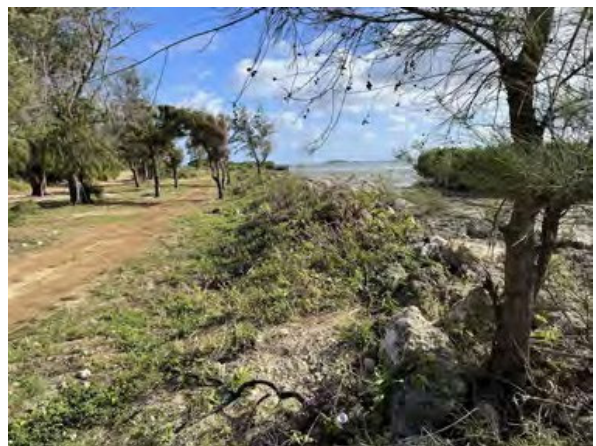
Photo 4.1.4 The height of seawall is lower
