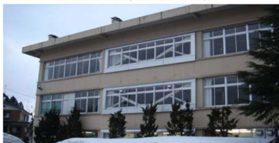
■ After reinforcement (exterior view)
