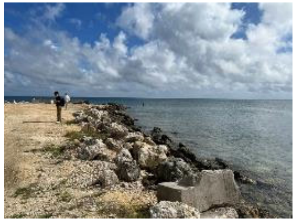
Photo 2.7.26 ②Length of seawall is about 130m
