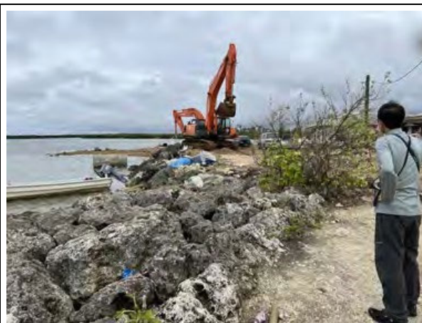
Photo 4.1.9 View facing east coast at the end of the coastal road
