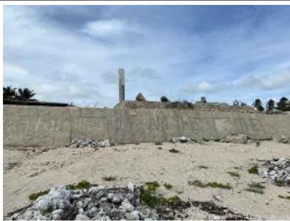
Photo 2.7.3 Foundation that Remained after a Tsunami
