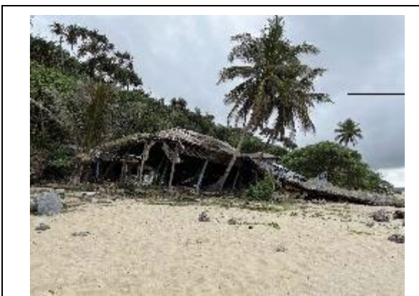
Photo 2.7.15 Resort Destroyed by Tsunami
