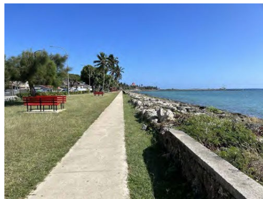
Photo 4.1.14 Collapsed part about 60m from left photo
