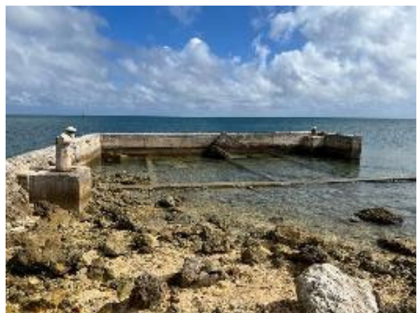
Photo 2.7.28 ④Caisson type mixed breakwater
