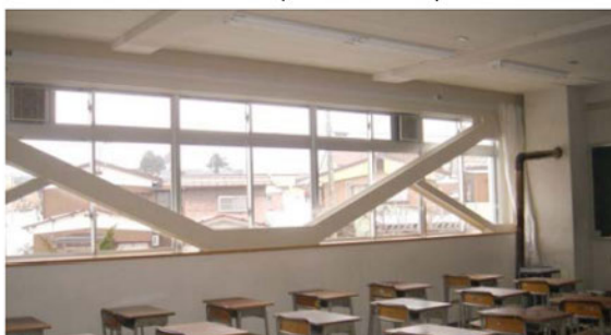
■ After reinforcement (interior view)
