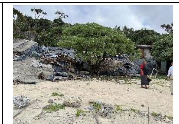
Photo 2.7.16 Resort Destroyed by Tsunami
