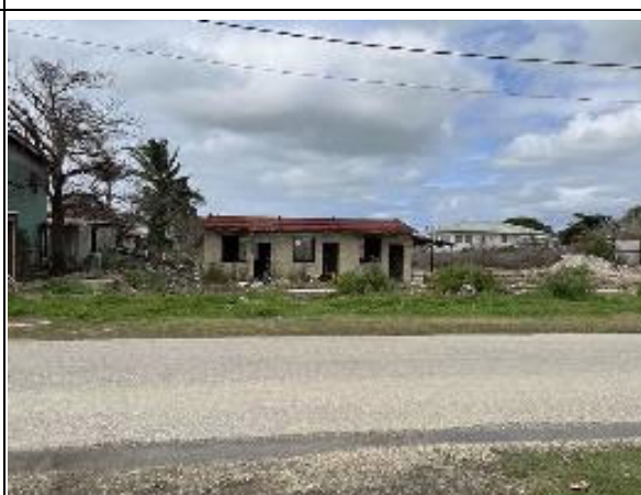
Photo 2.7.10 House Parts Washed away by Tsunami
