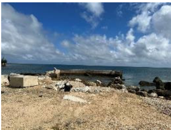
Photo 2.7.27 ③Tip of north wharf
