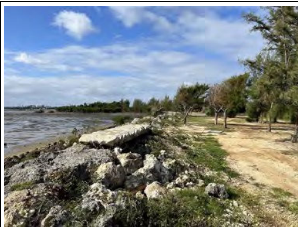
Photo 4.1.3 Restoration by casually piling up stones
