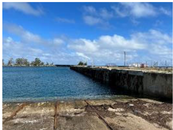
Photo 2.7.30 ⑥Sheet pile wharf from the ramp
