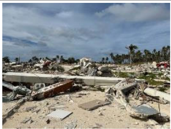
Photo 2.7.4 Completely Destroyed Resort Hotel
