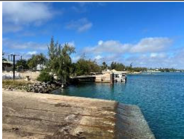
Photo 2.7.31 ⑦View of the jetty from the ramp
