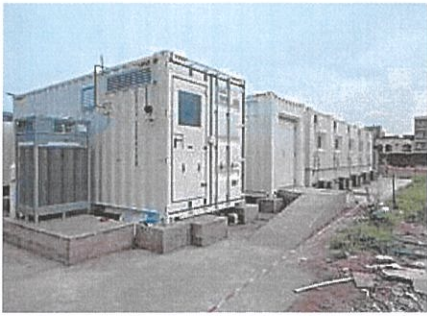
Exterior Panoramic View(South)
