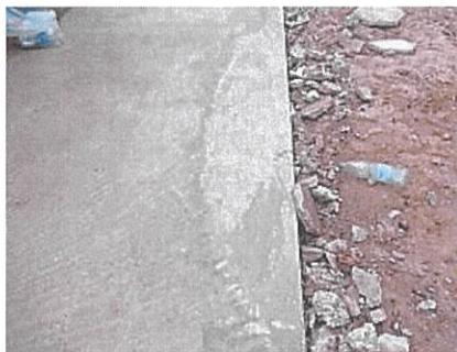
Concrete Slab Crack ⑦ (East Side)
