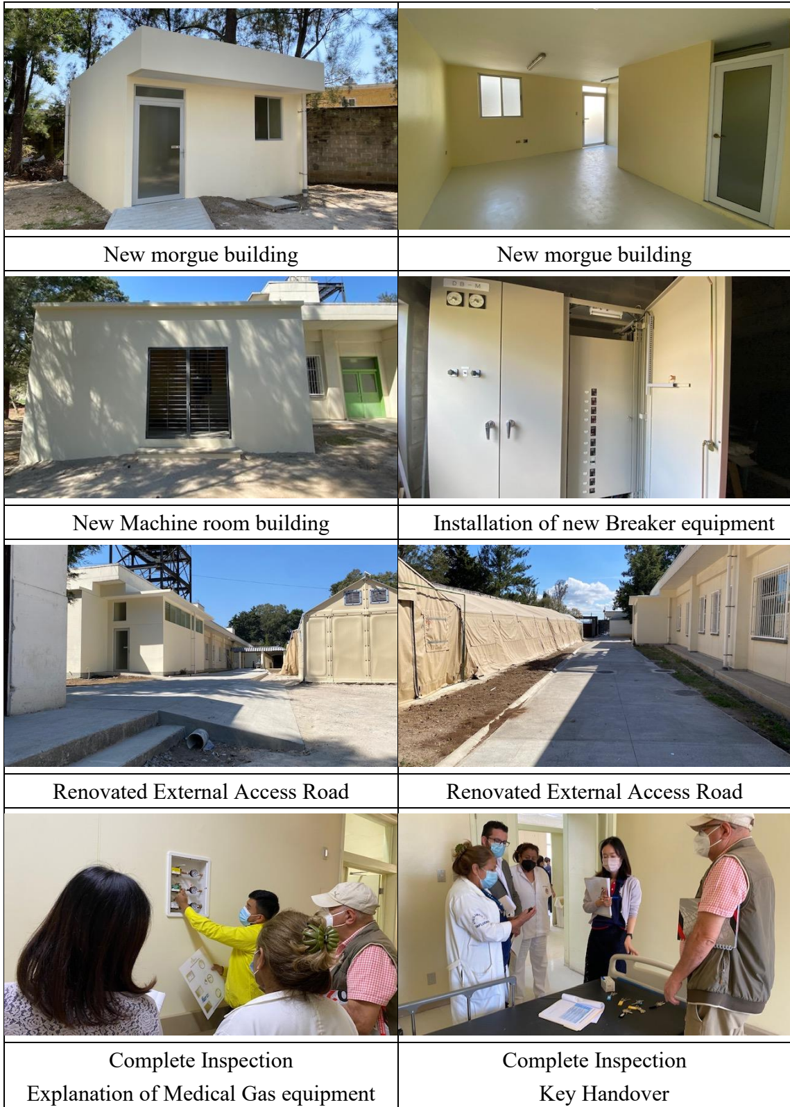
Figure3. Inspection of renovation works
