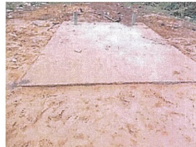
Concrete Slab Crack ⑧ (West Side)
