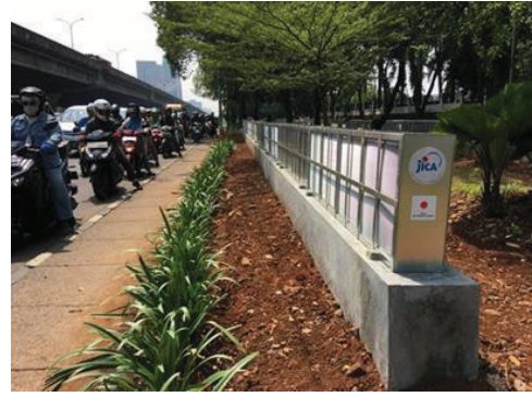
ACF Air Purification Units at the roadside (Jakarta, Indonesia , 2018)
