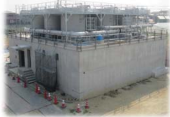
Medium scale municipal water supply (16,000 m 3 /day)
