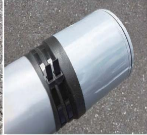
3 Apply tie band to prevent back rush.
