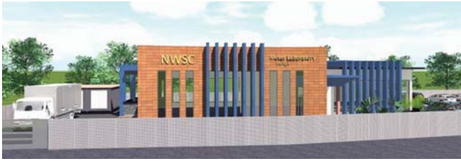
Modern Meter Laboratory and Meter Assembly Plant
