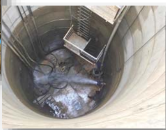
Radial Well Construction
