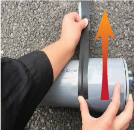
1 After taking backpaper, apply tensor to Tomezo, cover the leak spot.
