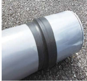
2 Wrap at least 3 layers or more to ensure stop leaks depending upon internal water pressure.
