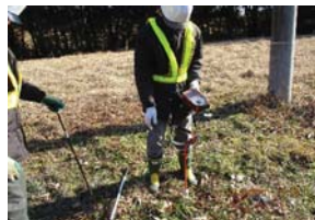
2. Tracing above buried pipe line with detector.
