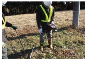
2. Tracing above buried pipe line with detector.
