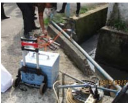
1. Injecting tracer gas
