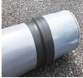
② Wrap at least 3 layers or more to ensure stop leaks depending upon internal water pressure.
