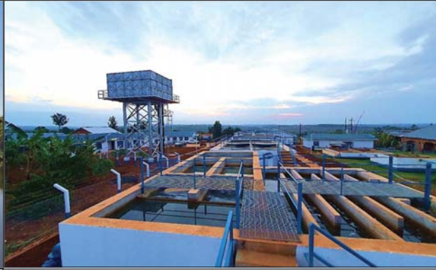
Sembabule Intake and Water Treatment Plant
