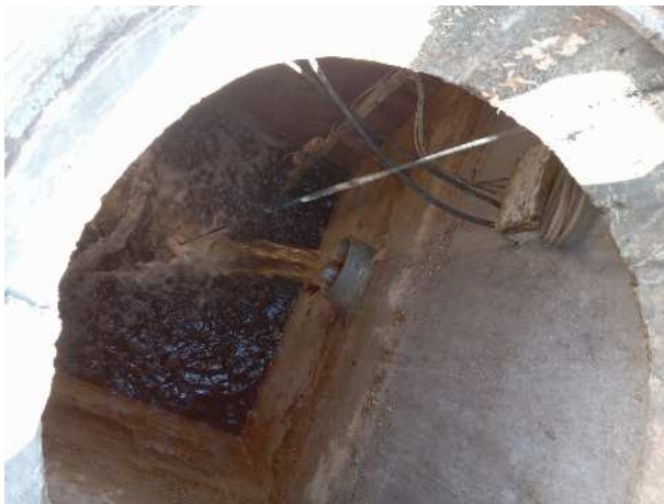
Inside the Septic tank
