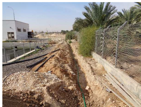
Photo 2.1.8 Construction of Power Lines
