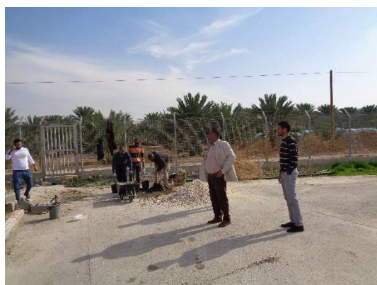
Photo 2.1.5 Mayor in WWTP (1)
