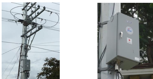
Figure 4.1 Testing for the commissioning
