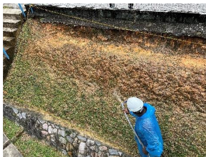
76. Site 2 Block A (from right side)
