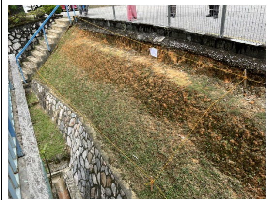
38. Site 2 Block A (from right side)
