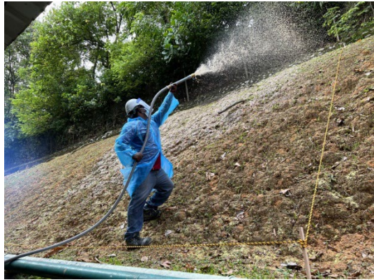
70. Site 1 Block B (from right side)
