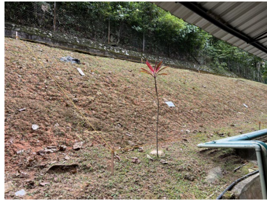
34. Site 1 Block C (from left side)
