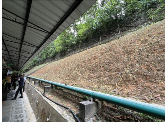
32. Site 1 Block B (from right side)
