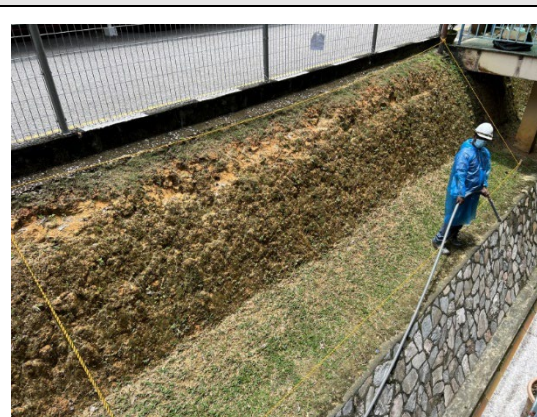
40. Site 2 Block B (from left side)
