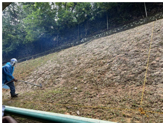
67. Site 1 Block A (from right side)
