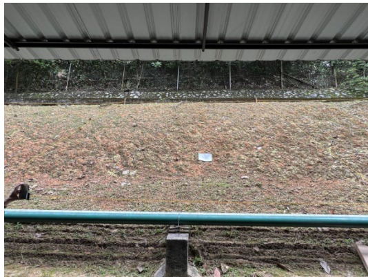
27. Site 1 Block A (front side)
