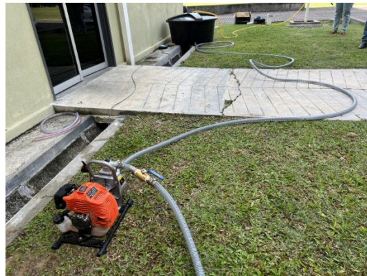
16. Tank to engine (from engine side to tank)
