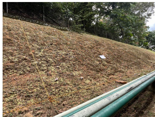
31. Site 1 Block B (from left side)
