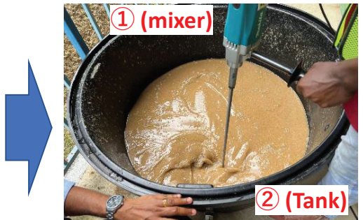
Mixing materials in the tank with water
