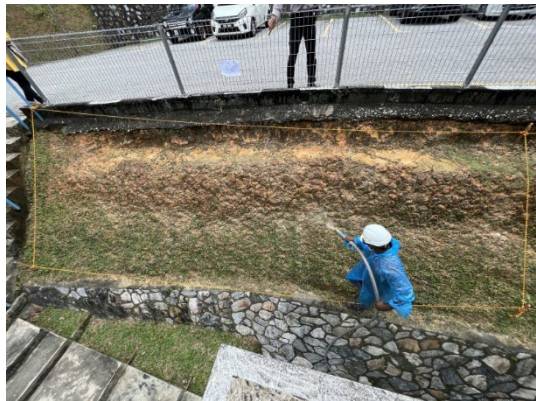
74. Site 2 Block A (front side)
