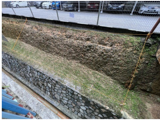
41. Site 2 Block B (from right side)
