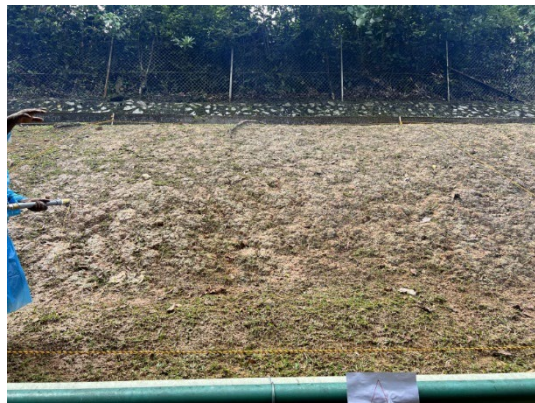
65. Site 1 Block A (front side)
