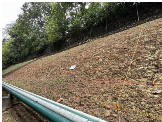
29. Site 1 Block A (from right side)
