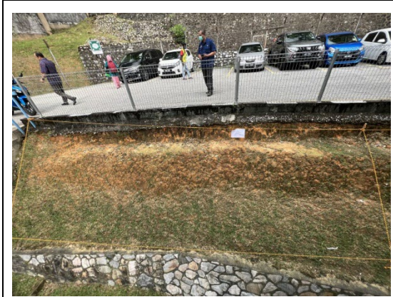
36. Site 2 Block A (front side)
