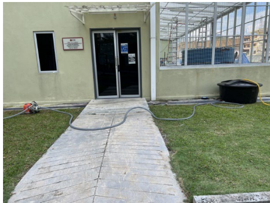
15. Tank to engine (front side)
