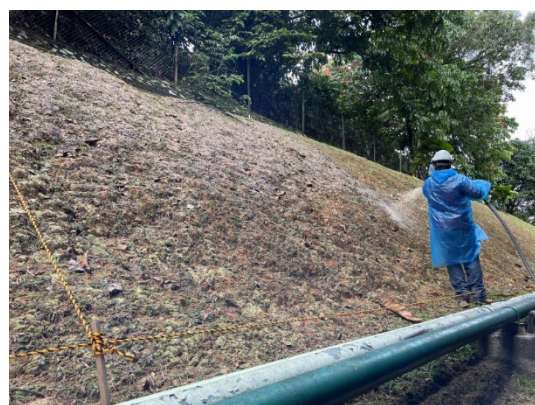
69. Site 1 Block B (from left side)
