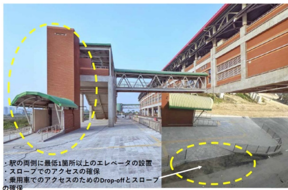
(i) Example of accessibility measures in station facilities: Elevators on both sides of the station and ramps
