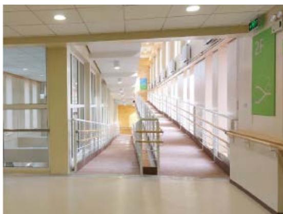
Gentle slope ramps for accessible buildings
