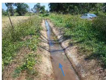
Right Bank Canal of Puliyan kulam
