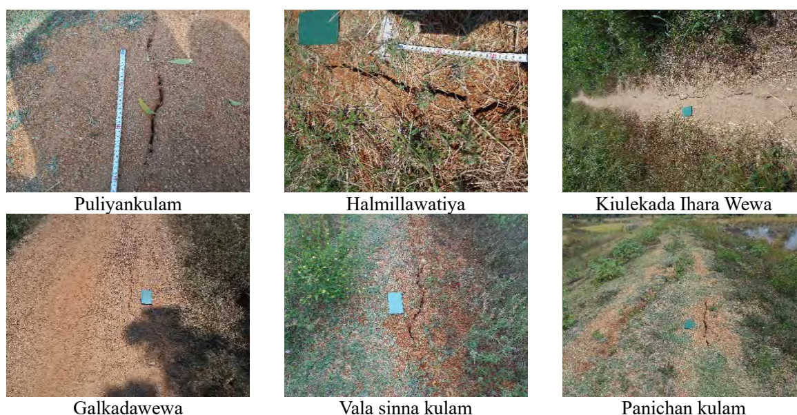
Figure 3.3-1 Cracks on Tank Bund
