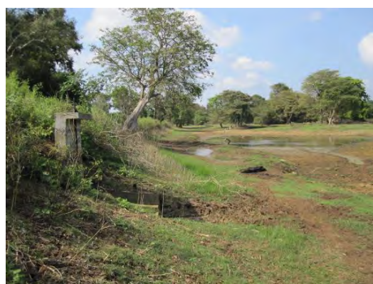
Overview of the Tank Bed and Sluice
