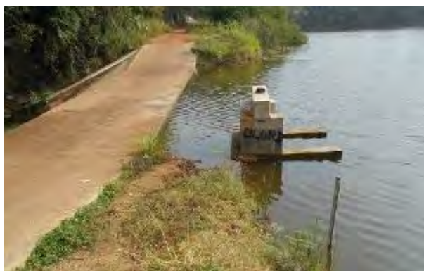
Pre-discharge Sluice Gate
