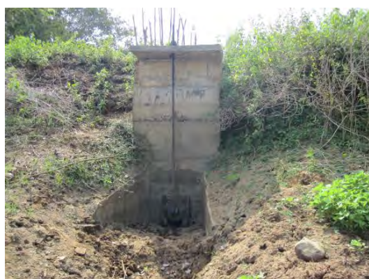
After Removing the Blockage of Inlet by Sedimentation
