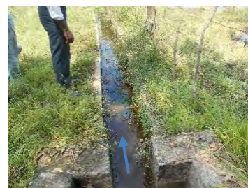
Left Bank Canal of Kakayar Puliyan kulam
