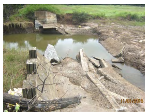
Figure 2.5-6 Flood Damage due to the 2014 Torrential Rains (Left: tank breach, Right: spillway collapse)
