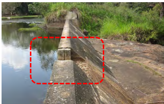
Spillway Wall Slit
