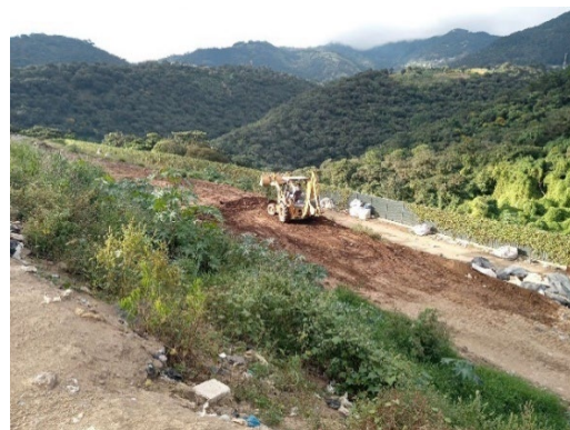
The status of compaction and covering at the same disposal site.
