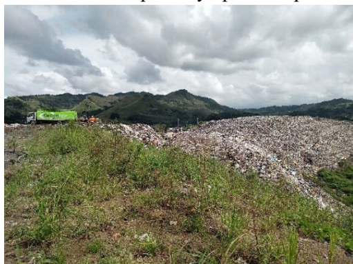
Cerro Patacon disposal site. Located on a slope, the site requires road maintenance for delivery of transportation trucks and heavy equipment.
