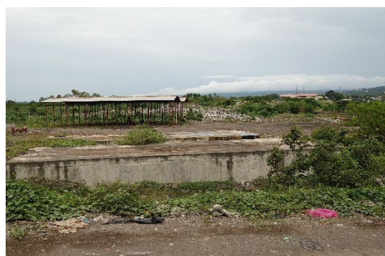
Water Treatment Facility at the Final Disposal Site in Managua City
