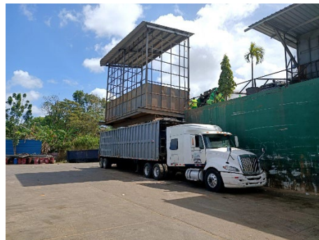
The waste brought in is transferred to larger trucks for transport to the disposal site.
