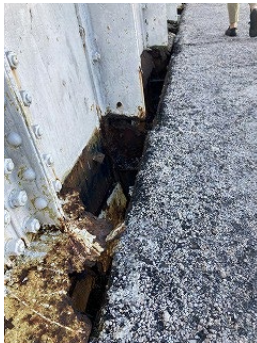
Figure 5-9 Steel Corrosion of Swing Bridge
