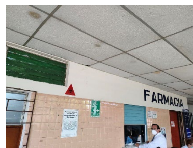
For the expansion of the radiology room, the pharmacy will be moved to another location. Another X-ray machine can be installed.
