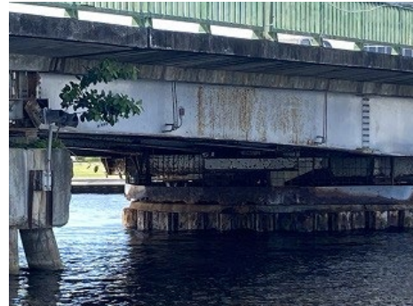
Figure 5-10 Belcan Bridge Pier (Corrosion of Pedestal)
