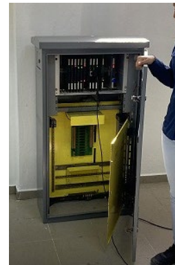
Figure 5-25 Remote Control Signal and Control Equipment
