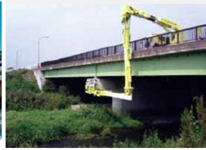
Bridge inspection example
