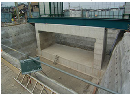
Hybrid Box Culvert
