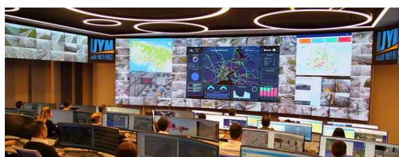
Traffic Control Center - Traffic and road network management
