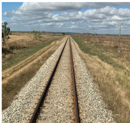
Central Line track
