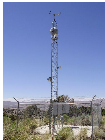
Road weather information system - Maintenance and construction management applications
