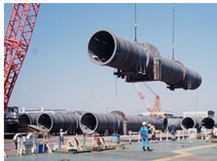
Water Pipe for Sea Water Exchanger
