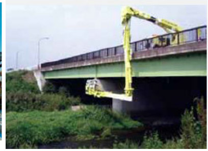
Bridge inspection example
