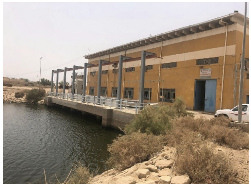
East Gharraf Drainage Pump Station
