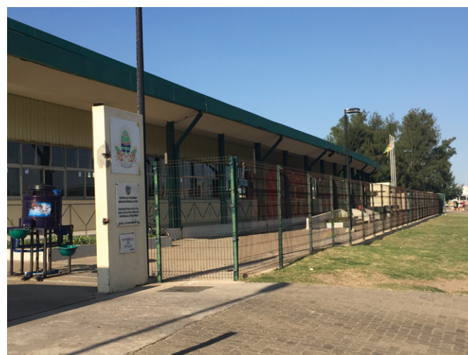
The exterior of Maputo Fish Market
