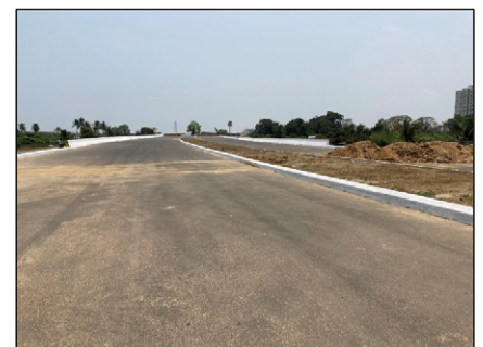
Small-scale infrastructure project under the Program (Construction of a bypass road)
