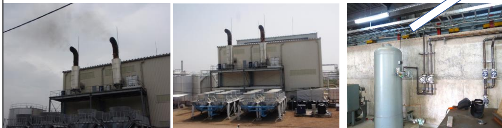
25% 1,250kW load condition 90% 4,500kW load condition on 12-2017
