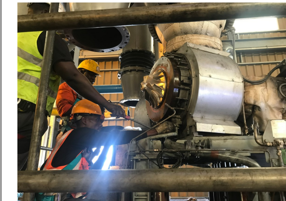
Overhaul Inspection of Turbocharger
