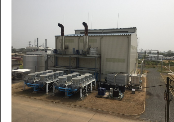
Power Plant (Exterior)
