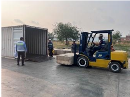
Loading concrete blocks
