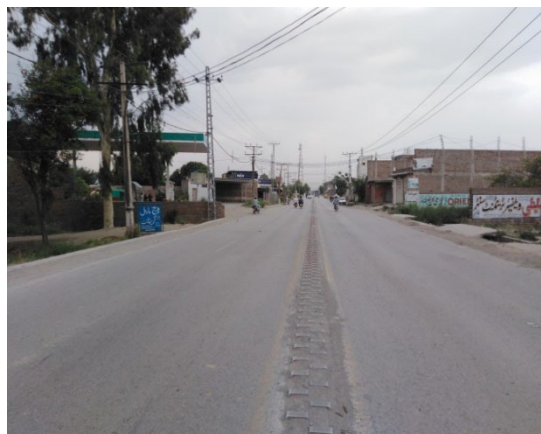
Provincial road after rehabilitation (Peshawar District)
