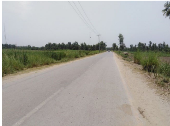
District road after rehabilitation (Mardan District)
