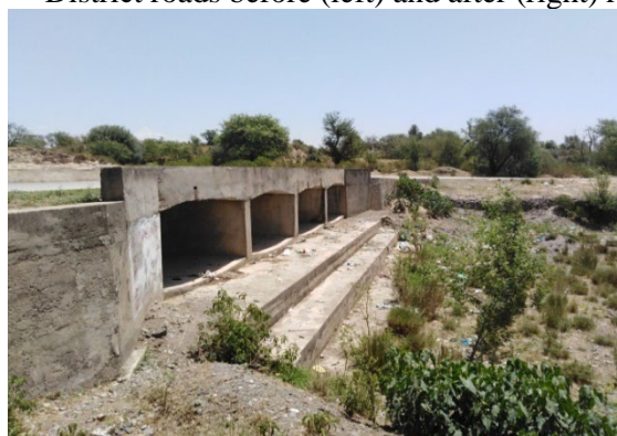
District road culvert after rehabilitation (Haripur District)
