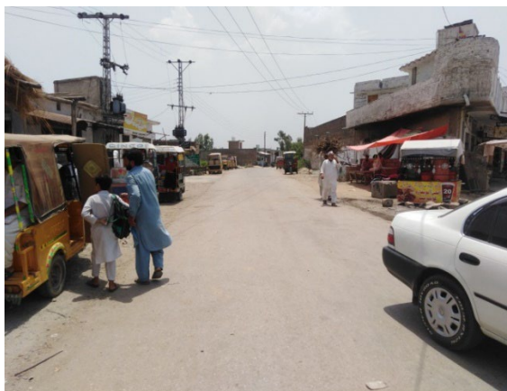
District road after rehabilitation (Mardan District)
