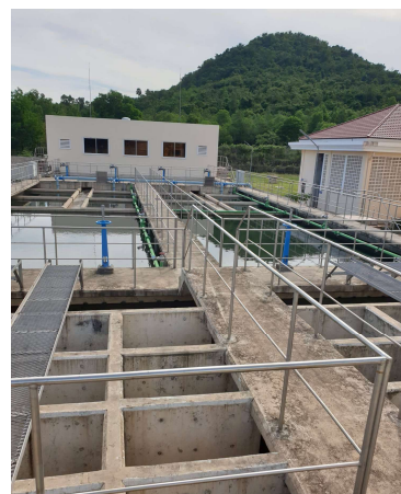
Sedimentation Basin at the Water Treatment Plant
