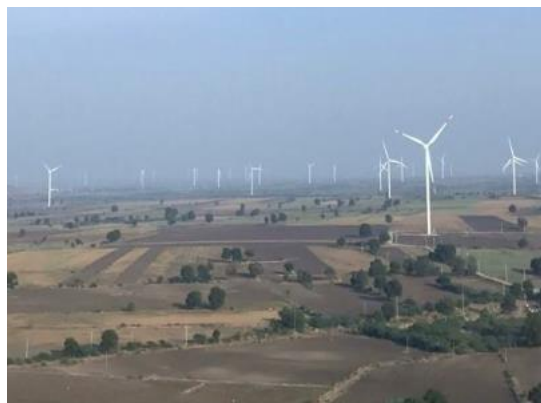
Wind power generation facility constructed by the Project (Source: Project materials prepared by the ACP investment team)
