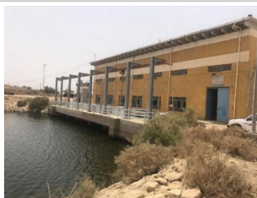
East Gharraf Drainage Pump Station (source: Ex-Post Evaluation Team 1 )
