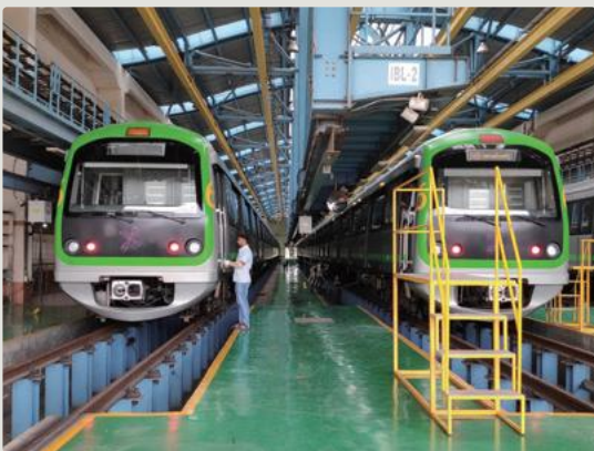
Maintenance at a depot
