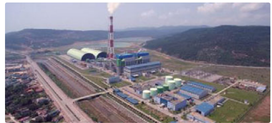
A panoramic view of the Power Plant (Nghi Son Thermal Power Plant Construction Project in Viet Nam)
