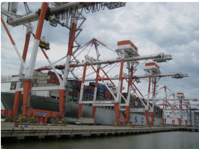
A berth and cranes in the Cai Mep container cargo terminal
