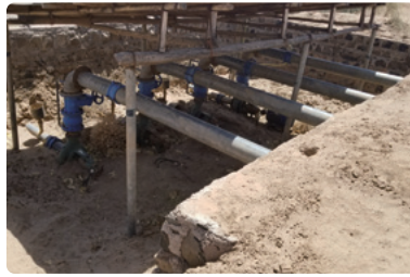
Irrigation facility constructed in Somali Region (Output 2)
