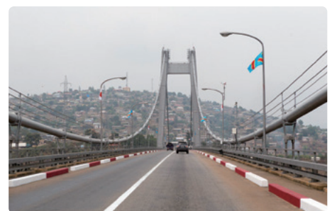
Main cables with the dry-air injection system installed. The city of Matadi located to the front. Photo taken by Shinichi Kuno
