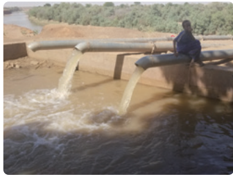
Irrigation facility constructed in Somali Region
