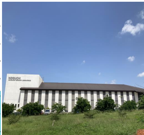
The whole view of ARC at NMIMR
