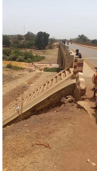
Falémé Bridge (Photo taken by the local assistant)
