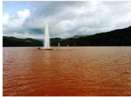
Deep lake water discharged from a degassing pipe installed in Lake Nyos
